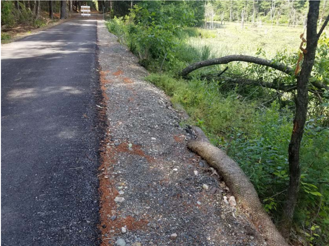
EROSION CONTROL TO BE PLACED
