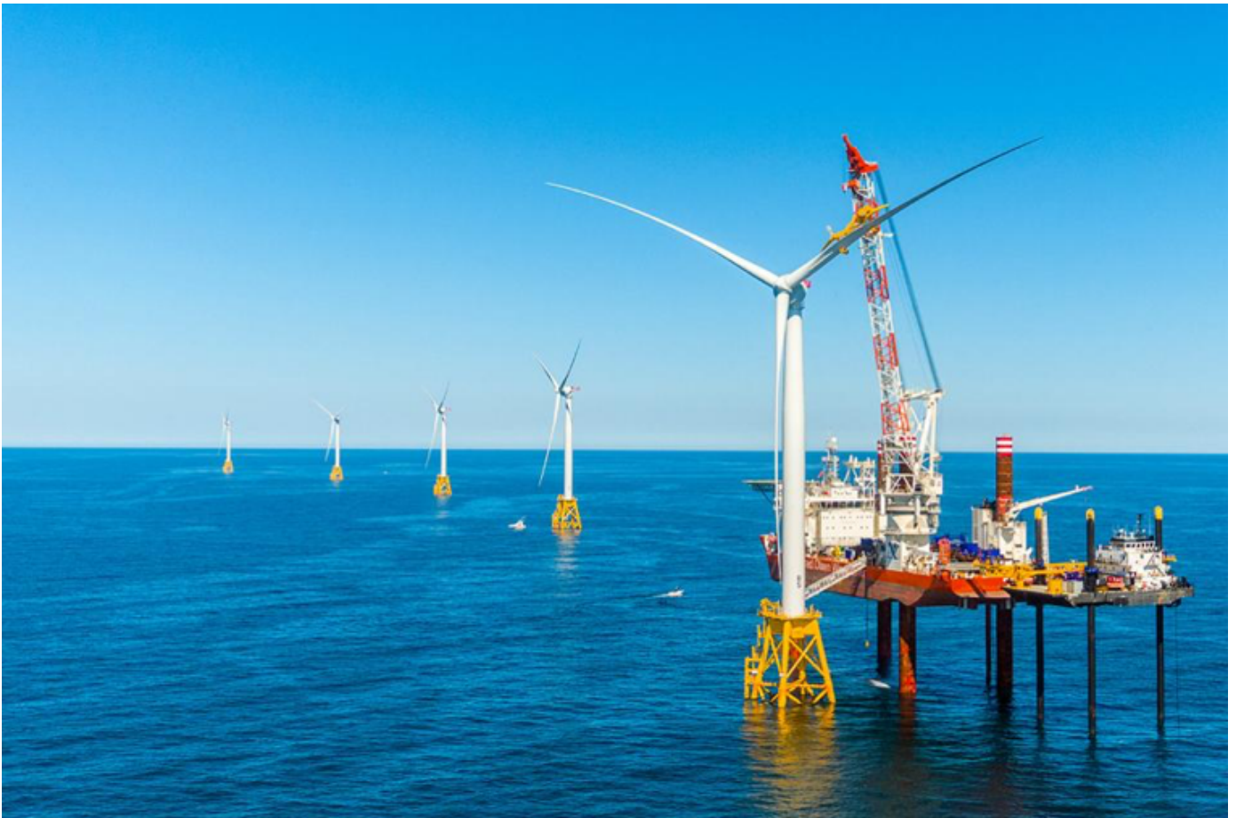
Block Island offshore wind farm construction
