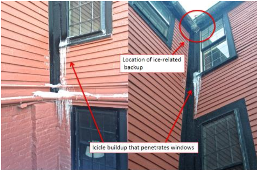
Figure 16: Gutter assembly – west elevation. (See also Figure 27.)
