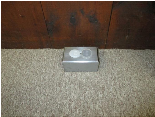
1 st : 6 South wall Room 108
