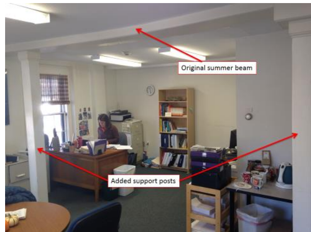
Figure 34: Room 109 showing original north-south summer beam with intact casing.
