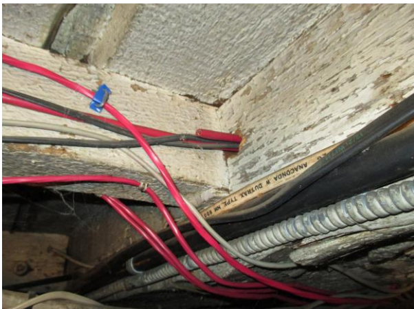
BAS: 26 Center bay, east side
