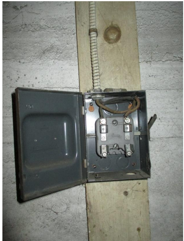
BAS: 23 Center bay, east side
