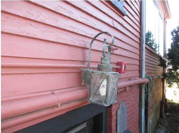
Ext: 16 West elevation of sun porch
