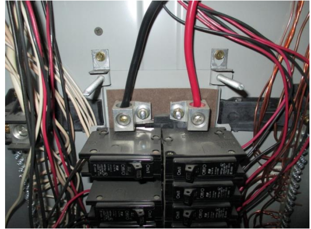
3rd: 8 South room
