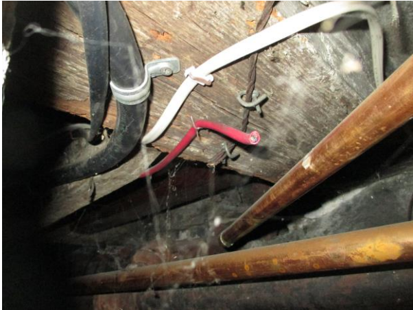
BAS: 24 Center bay, east side
