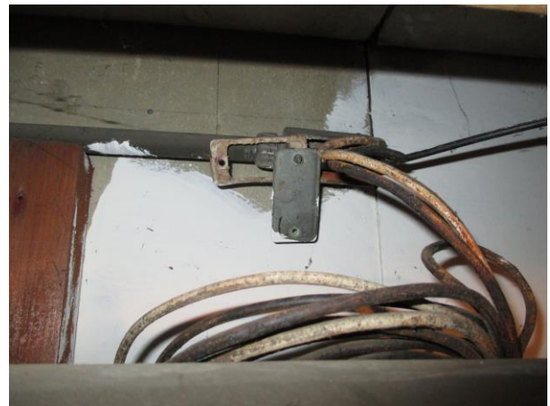
BAS: 18 Center bay, east side.
