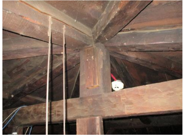
Figure 49: View of upper (unfinished) attic showing construction details.
