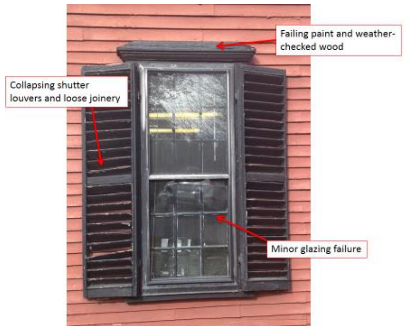
Figure 12: Typical shutter and window conditions.
