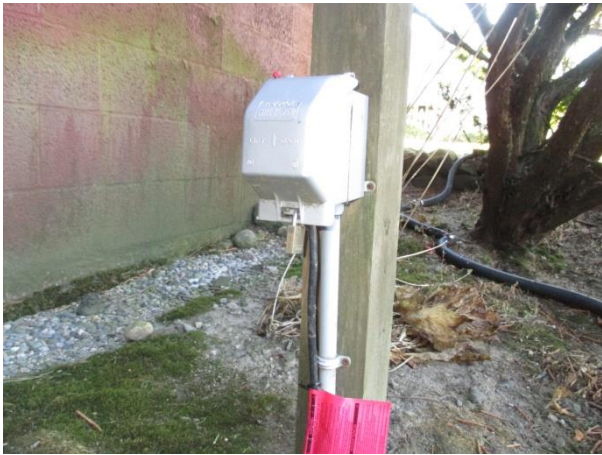
Ext: 17 West elevation of sun porch
