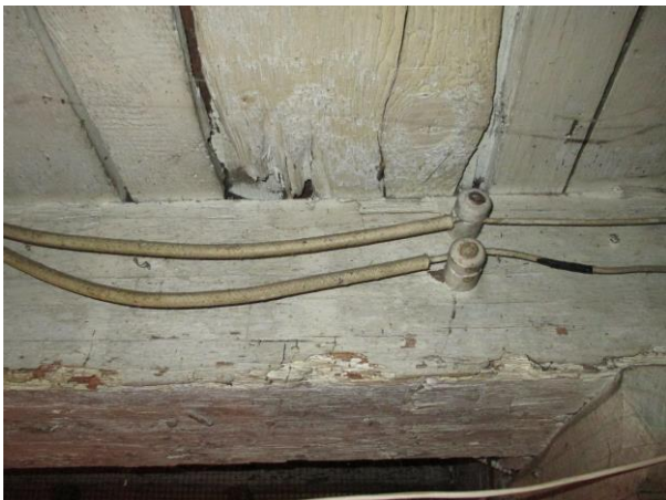
BAS: 21 Center bay, east side
