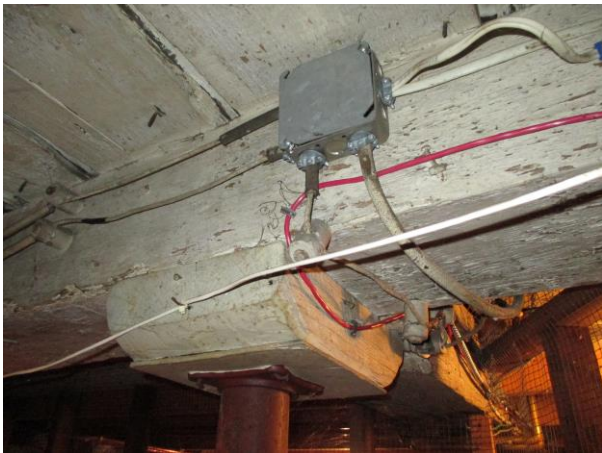
BAS: 20 Center bay, east side
