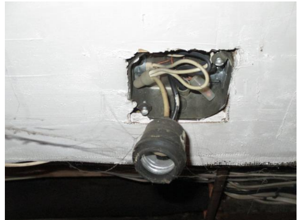
BAS: 9 Center basement ceiling
