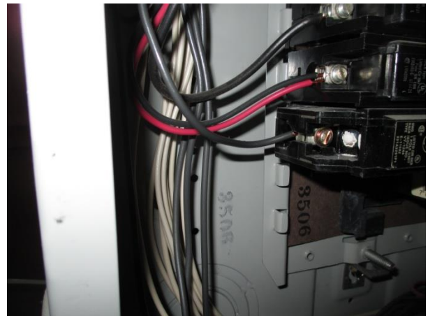
3rd: 10 South room
