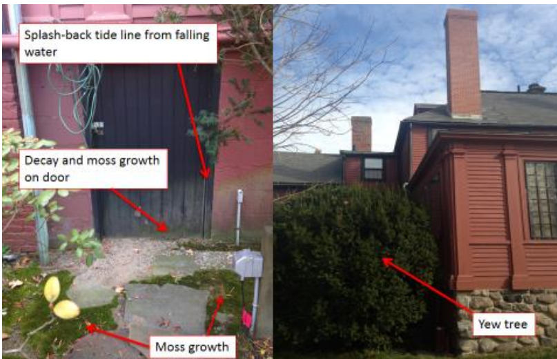
Figure 17: Two views of the west elevation showing encroachment of the yew tree and the effects of trapped moisture.
