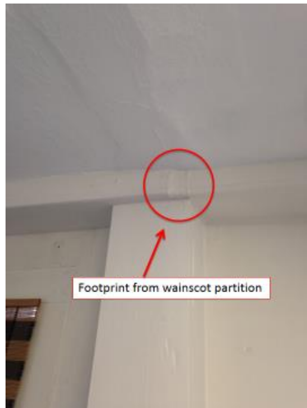
Figure 36: Room 109, intersection of the west wall girt and post showing evidence of an earlier wainscot wall partition.
