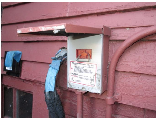
Ext: 13 South wall
