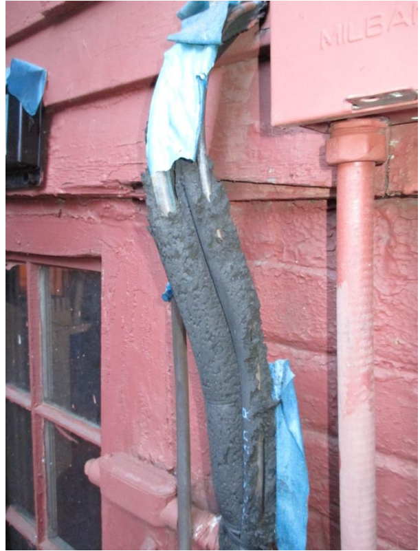
Ext: 14 South wall
