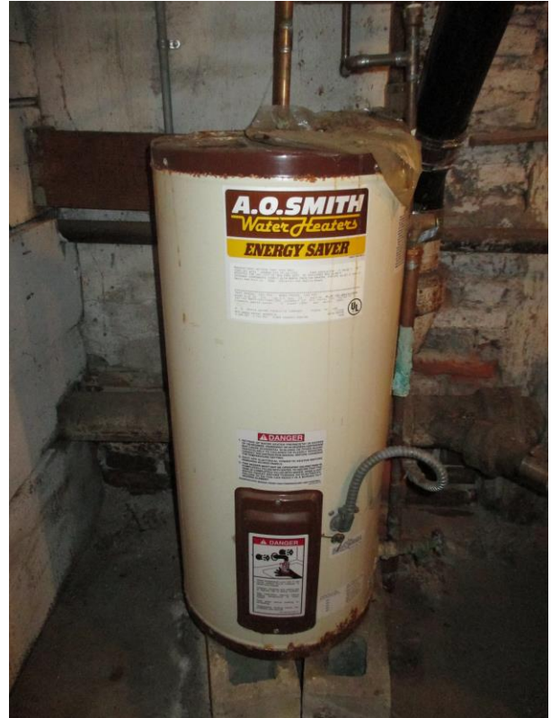
BAS: 27 Center bay, east side
