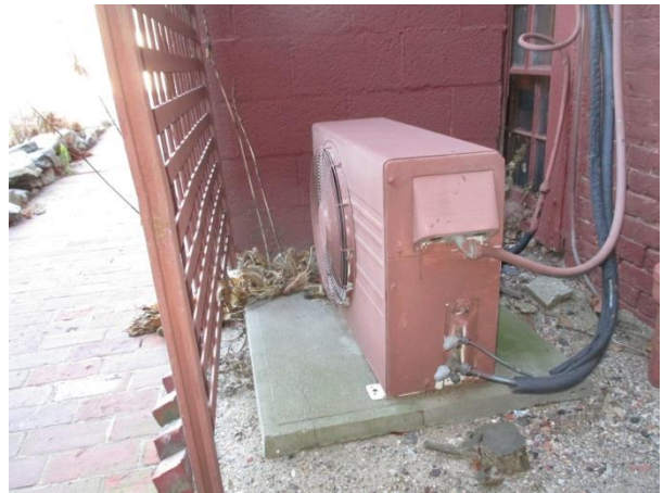
Ext: 15 South wall
