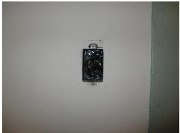
1 st : 4 West wall Room 103
