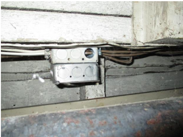
BAS: 25 Center bay, east side
