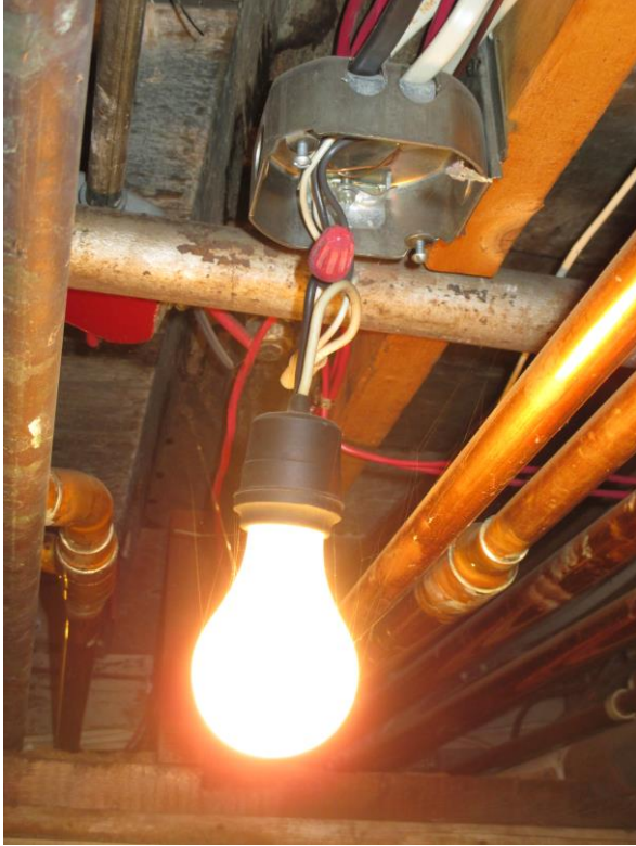
BAS: 10 Center basement ceiling
