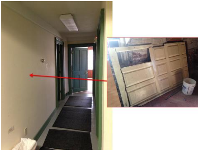
Figure 22: View of south hallway looking south. The fielded paneling stored in the basement may originally have been located on the east wall of 100c.
