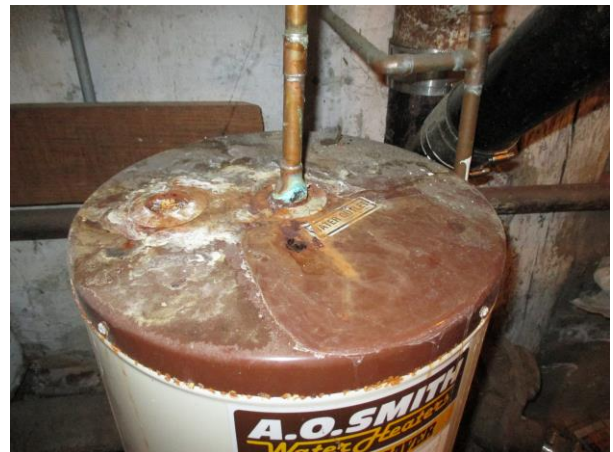
BAS: 28 Center bay, east side
