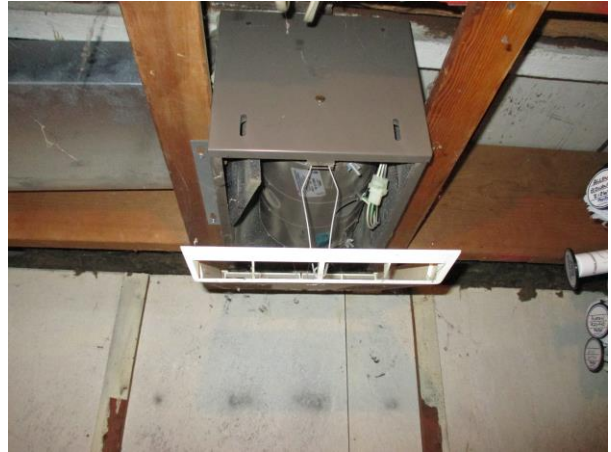
BAS: 22 Center bay, east side
