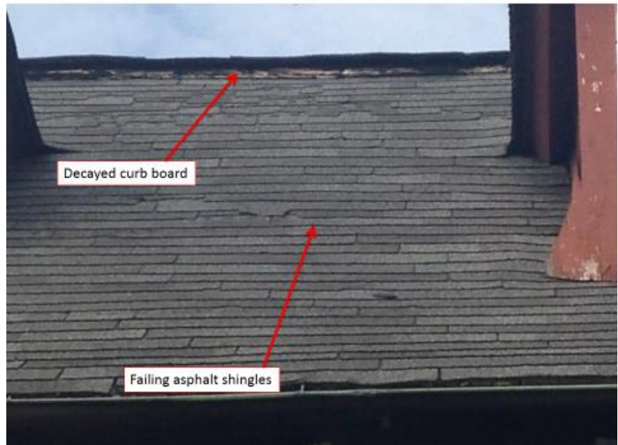
Figure 14: Typical roof conditions.
