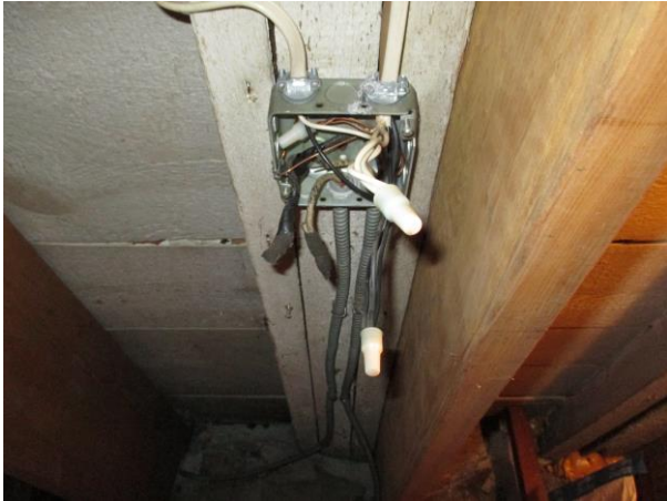
BAS: 19 Center bay, east side
