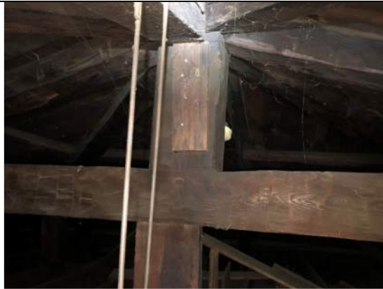
3) Center post in attic above ceiling.
