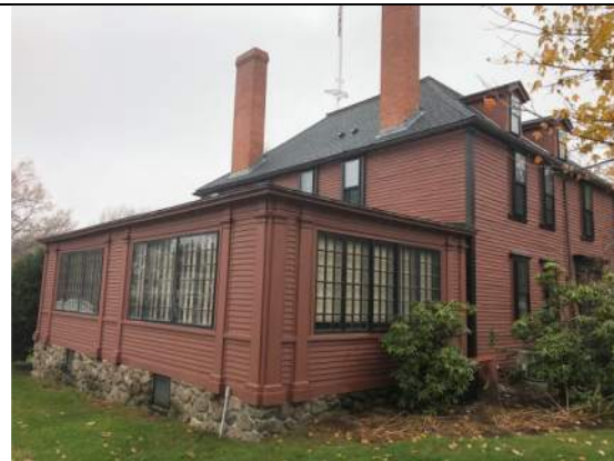
2) South west elevation, area 3 single story area in foreground.
