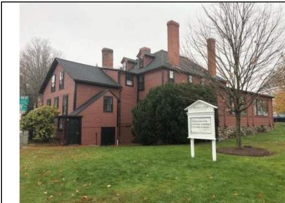
1) North west elevation, area 2 to left, area 3 to right and area 1 center.
