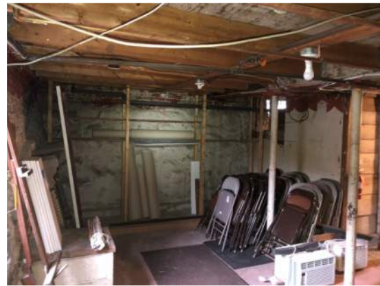
20) General first floor framing in area 2.
