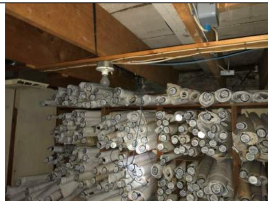
24) Sample floor joist sisters in area 1 with inadequate support at foundation wall.
