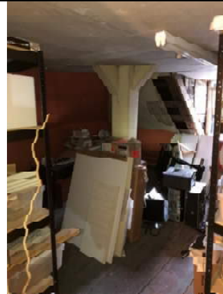
6) Continuation of hip post through third/attic level.
