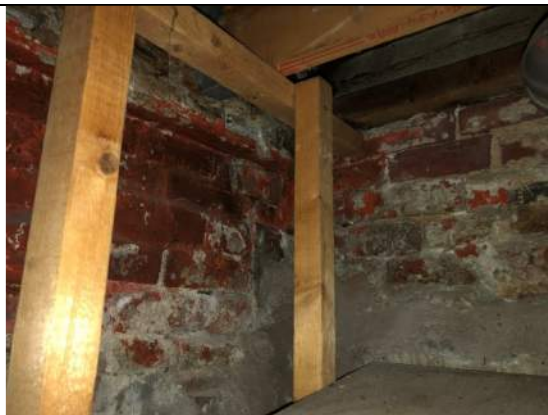
27) Interior side of wall at photo 28, no crack visible.
