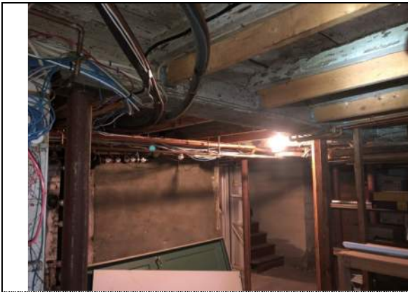
25) General first floor framing of area 1.
