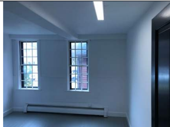
16) Exposed second floor timber beams in ceiling of first floor.
