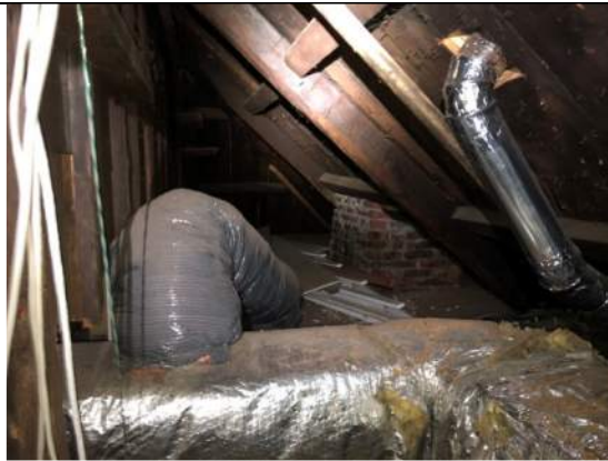
9) Sagging rafters on west facing hip roof of the original 1747 construction in area 1.
