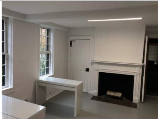
15) Exposed second floor timber beams in ceiling of first floor.
