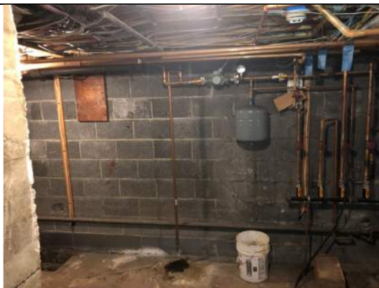
23) Concrete masonry wall along center line in area 1 and beneath center post to roof.
