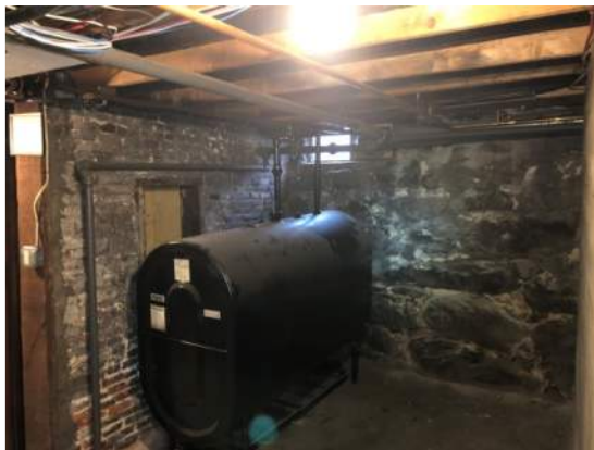
21) General condition of field stone wall and interior brick masonry walls.
