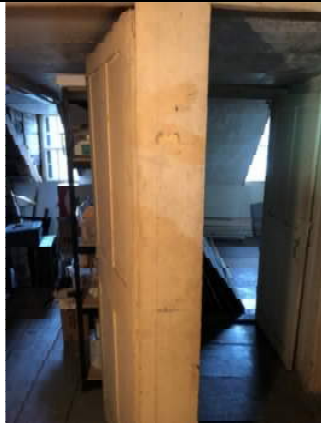
5) Continuation of center post through third/attic level.
