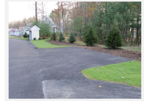
Powder Mill Woods Parking Area
