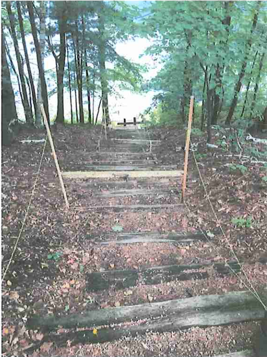
Steps to be replaced (facing White Pond)
