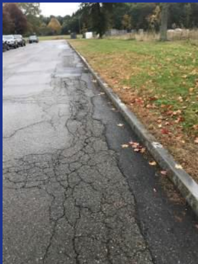
Multiple patches and significant cracking
