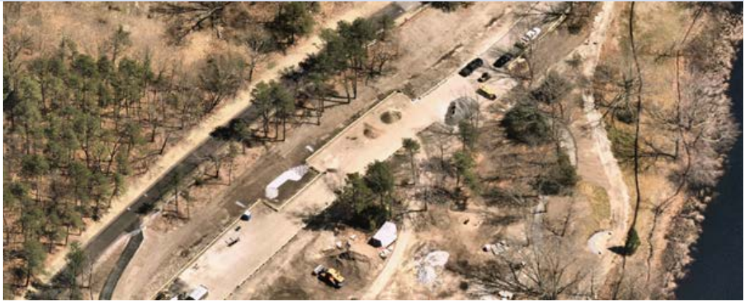
Gerow Recreation Area - work in progress
