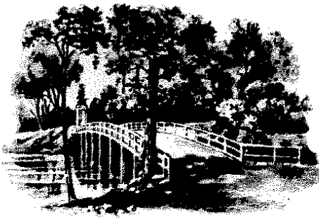
OLD NORTH BRIDGE
