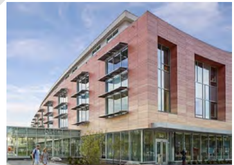
Figure 1. The Cambridge King Open and Cambridge Street Upper School Campus is Net Zero Ready (Photo by Robert Benson) www.mma.org
