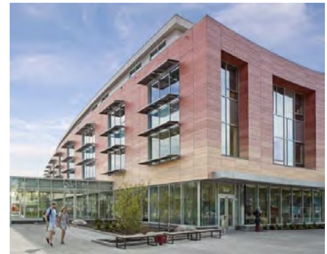
Figure 6. The Cambridge King Open and Cambridge Street Upper School Campus is Net Zero Ready (Photo by Robert Benson) www.mma.org
