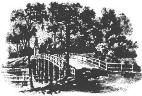
OLD NORTH BRIDGE
