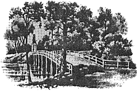
OLD NORTH BRIDGE
