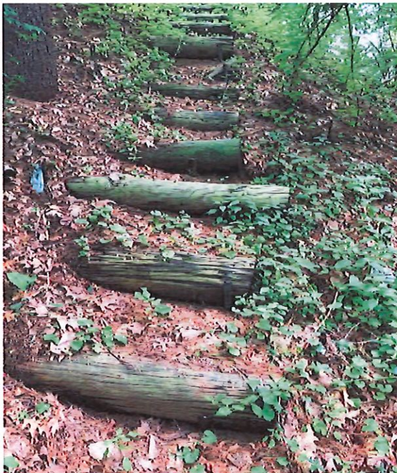
Figure 4: View of stairs from bottom of hill
