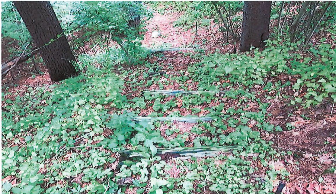
Figure 2: Bottom section of stairs
