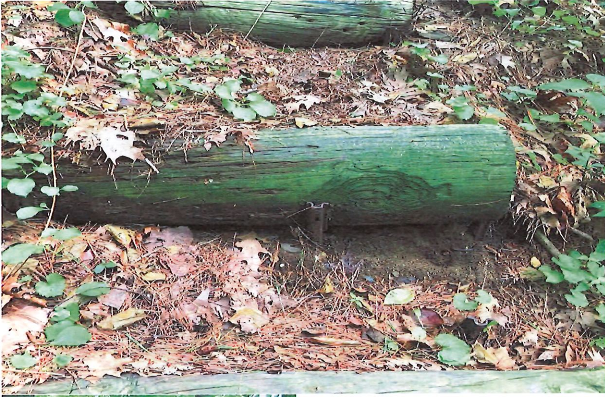
Figure 3: Step dug into hillside and secured in place by metal post
