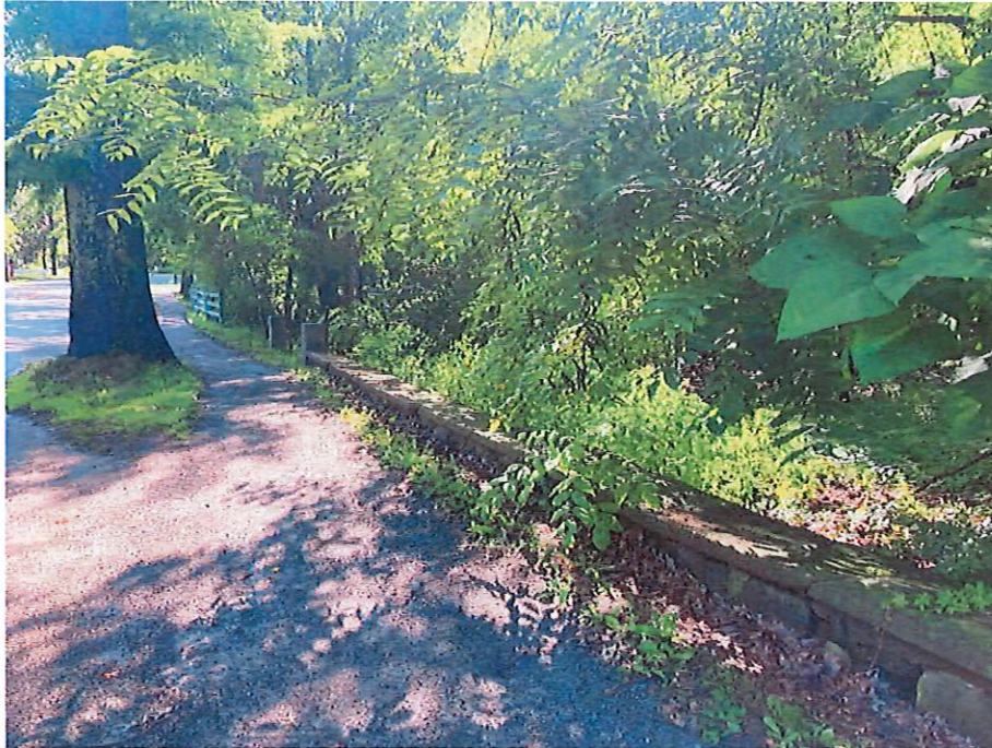
Figure 1: Wall to be restored
