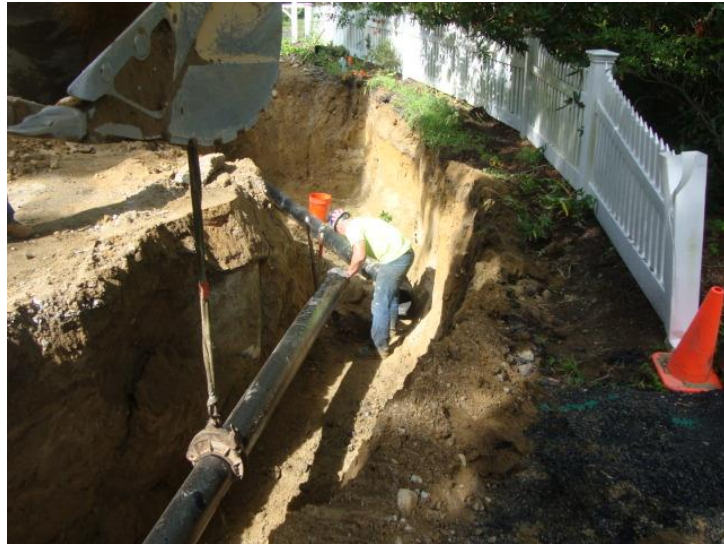
Southfield Road Water Main Project
