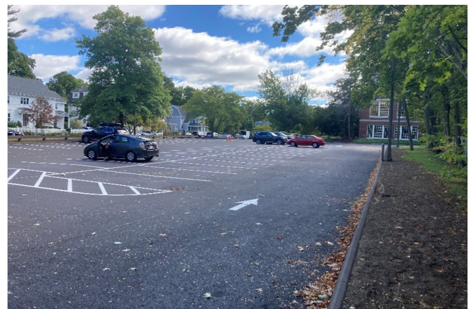
Stow Street Parking Lot Reconstruction Completed
