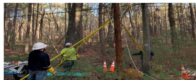
Hand Setting Poles Fairhaven Wood and MASSPORT Hanger Project Virginia Road
