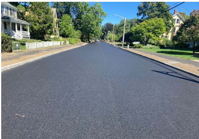
Hubbard Street Final Paving
