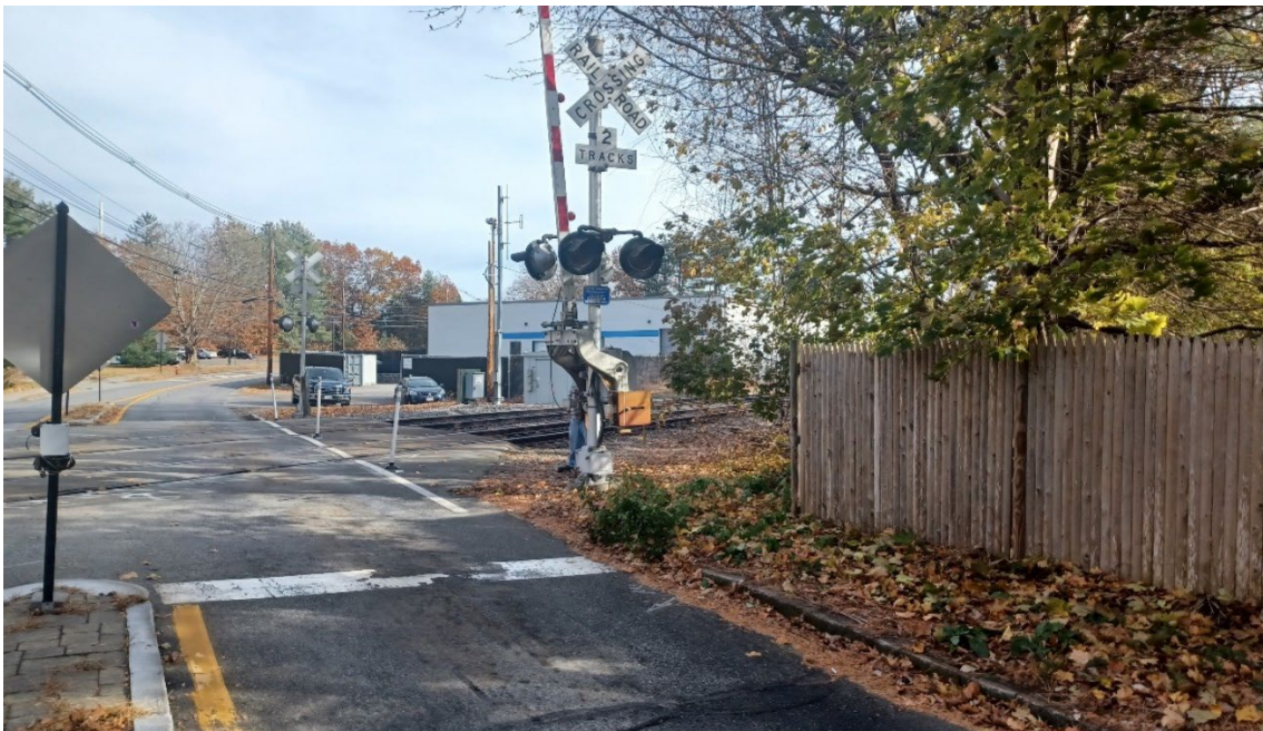
Photo 8: Crossing view of southeast quadrant
