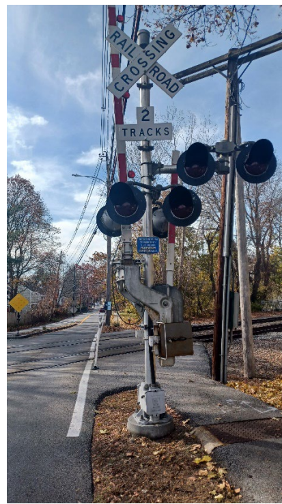
Photo 11: Signal on northwest quadrant, showing pedestrian gate geared to same mechanism as roadway gate
