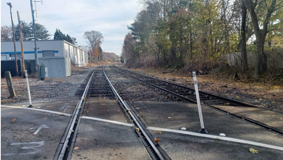
Photo 5: Track from crossing, view east
