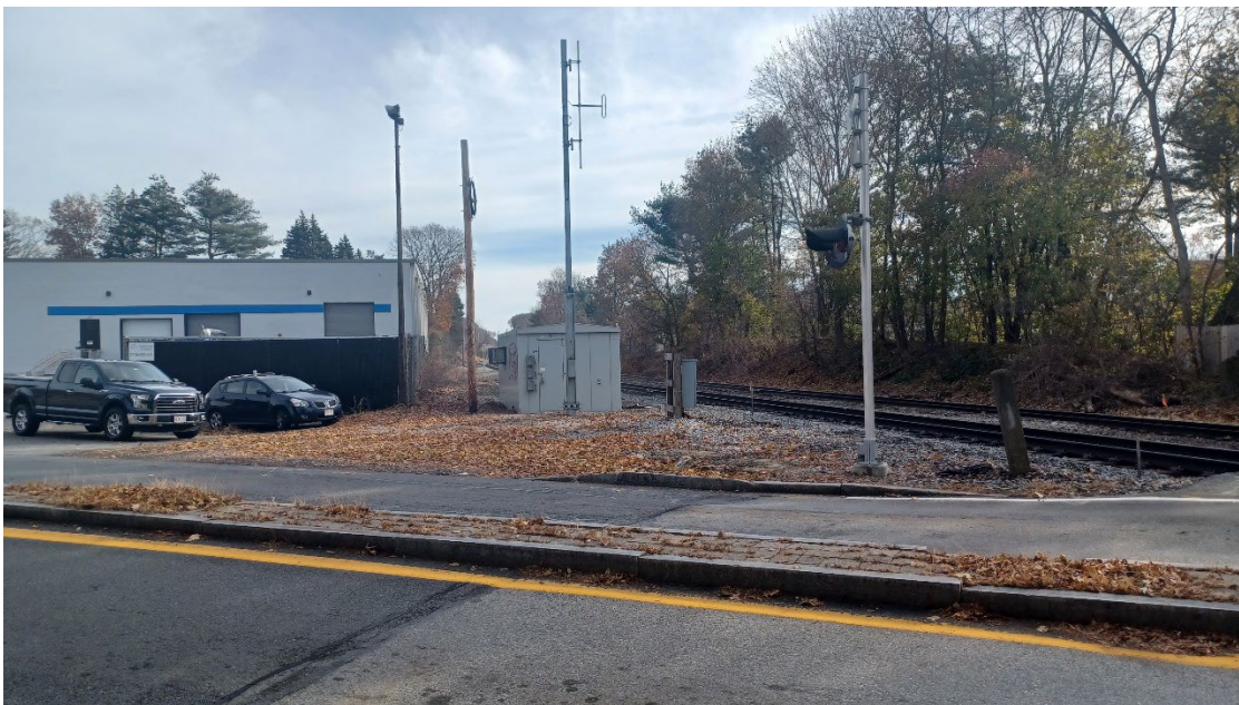
Photo 4: Limited/Obstructed view of approaching trains, seen from north side of crossing, looking east.
