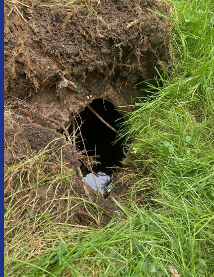
Minot Rd – Collapsed pipe, Root-Clogged pipe
