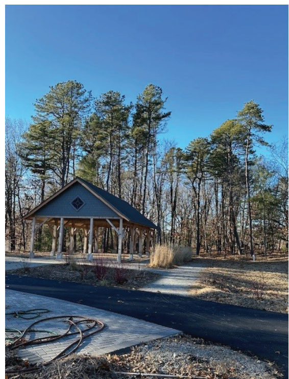
Completed Pavilion Structure
