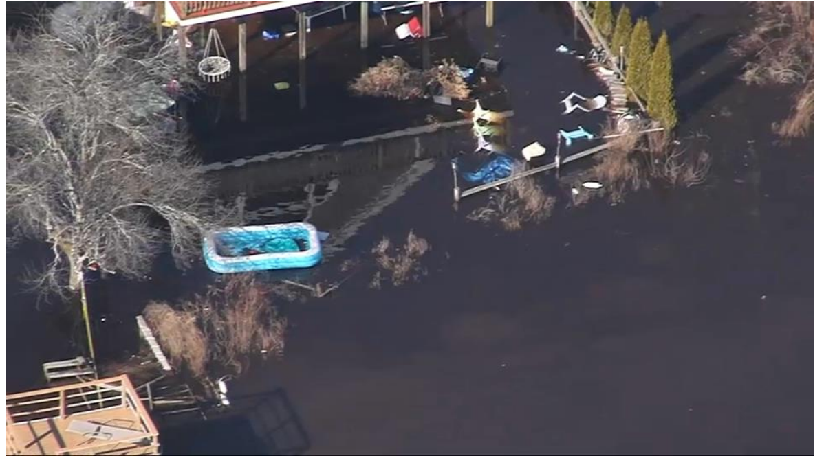
Dam Breach flooded back yards in Bridgewater-Image Credit WBZ Boston
