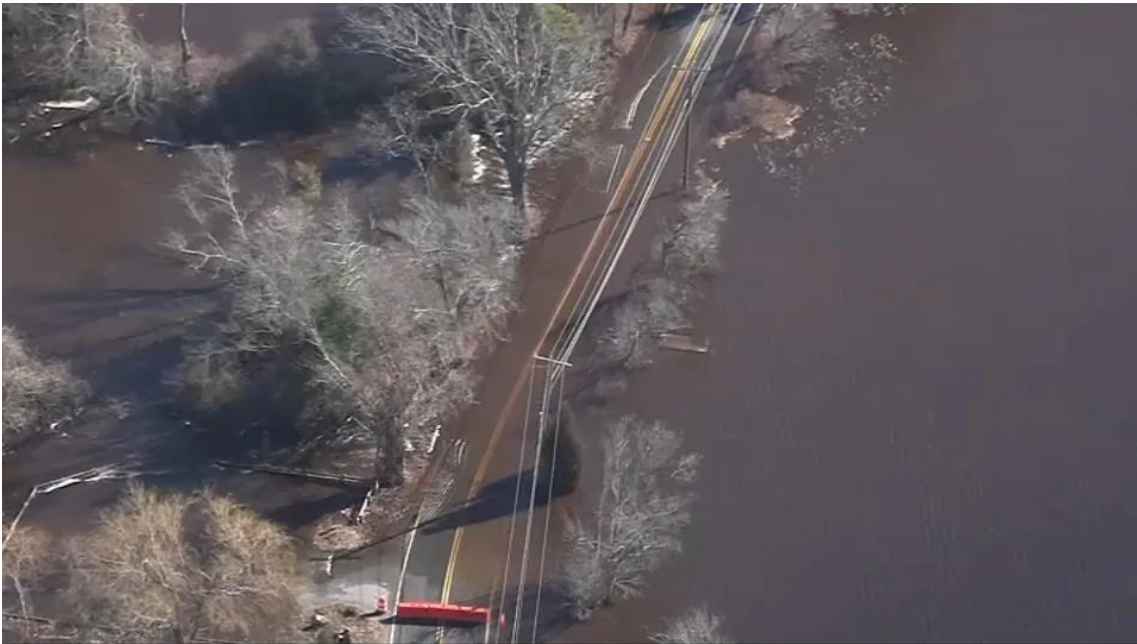
Dam Breach flooded road downstream in Bridgewater Image Credit: WBZ Boston
