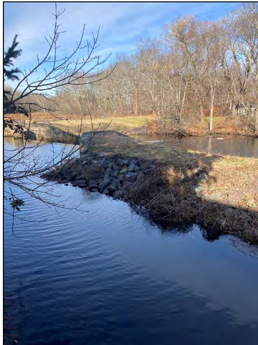
Photo No. 23.: Overview of the upstream slope between spillways and downstream slope left of the primary spillway post clearing (Provided by Town 2023-11-29).
