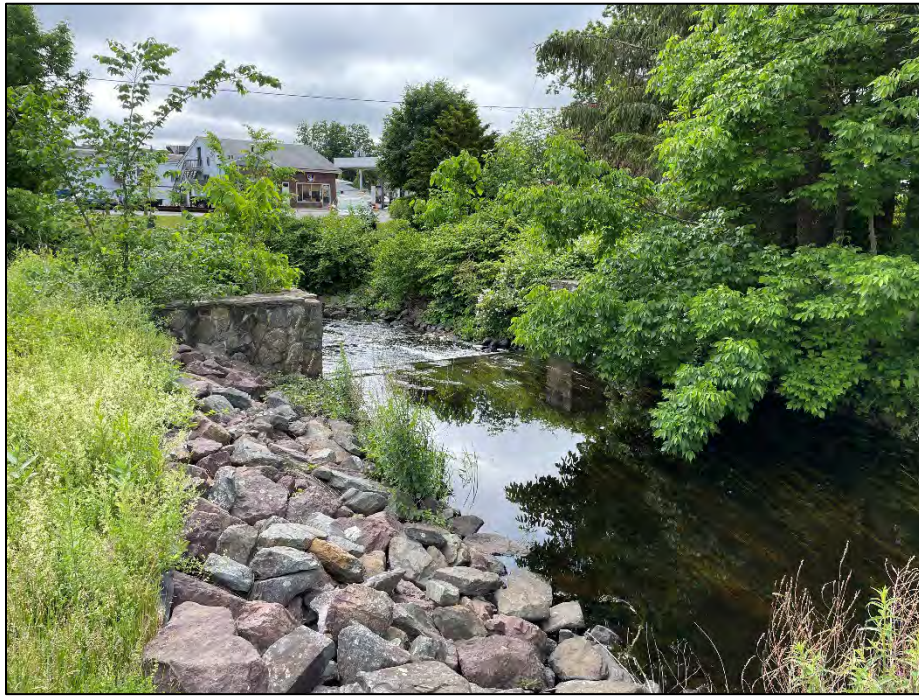
Photo No. 17.: Upstream side of the auxiliary spillway
