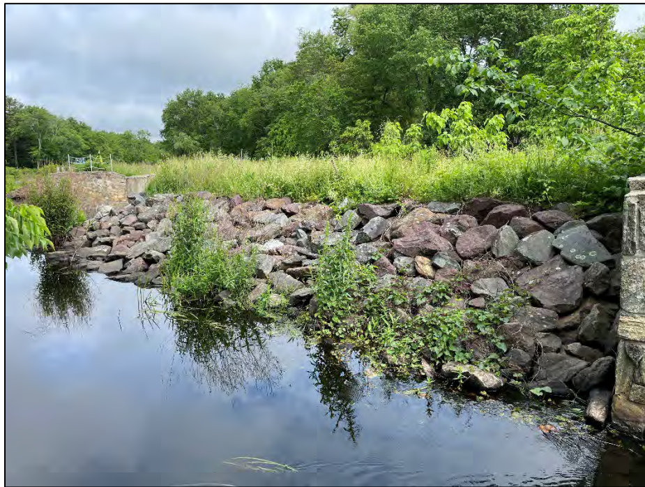
Photo No. 8.: Upstream slope of the embankment between the spillways
