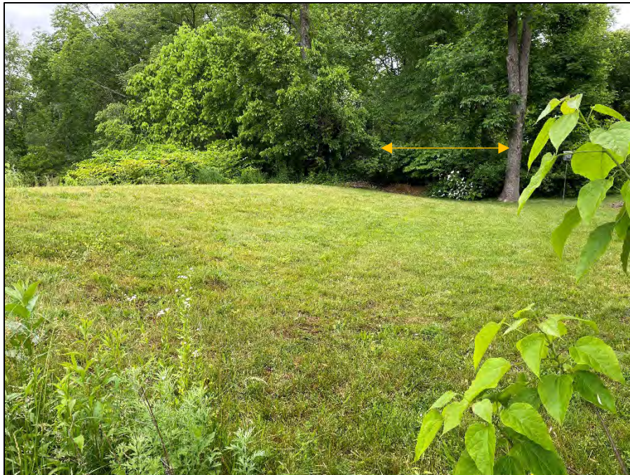
Photo No. 4.: Crest and downstream slope near 0+50 looking left. Note the apparent lower left abutment
