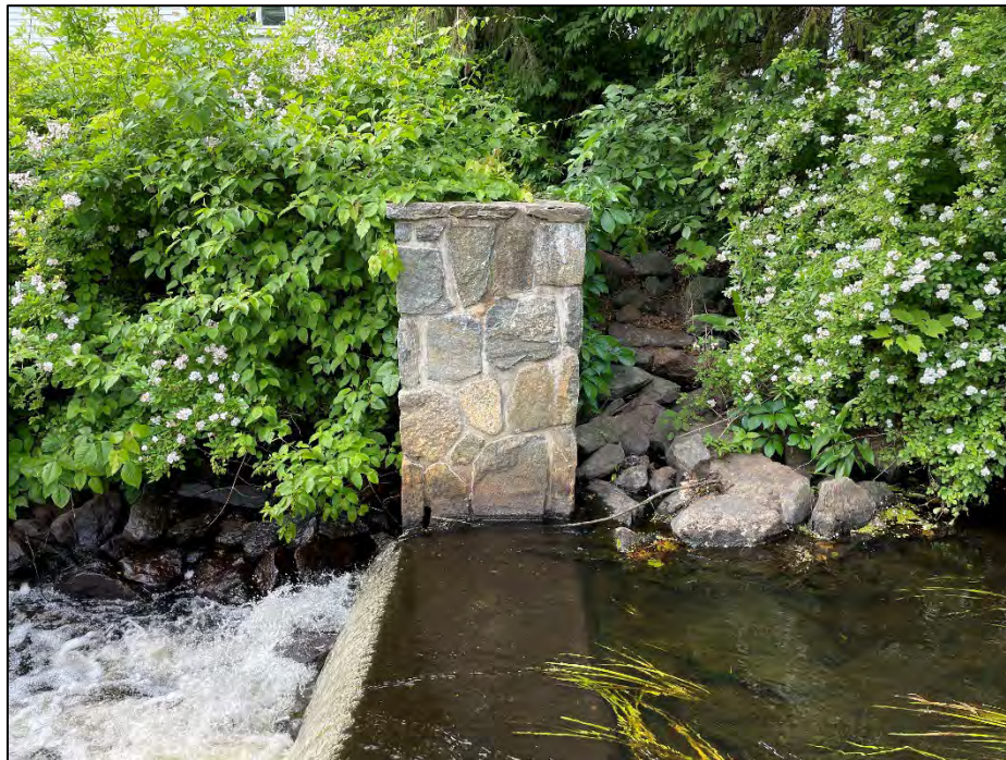
Photo No. 18.: Auxiliary spillway weir and right training wall
