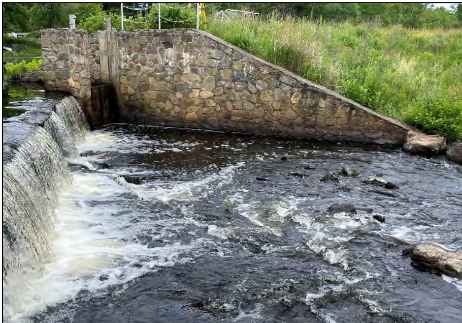
Photo No. 14.: Left training wall of primary spillway / sluiceway
