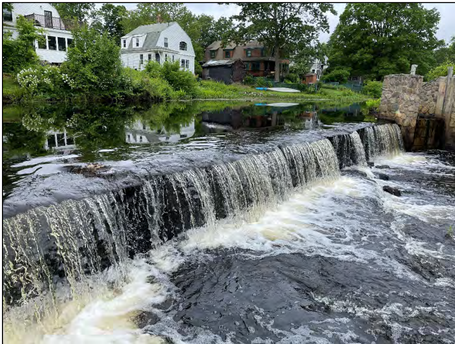
Photo No. 12.: Downstream side of the primary spillway.
