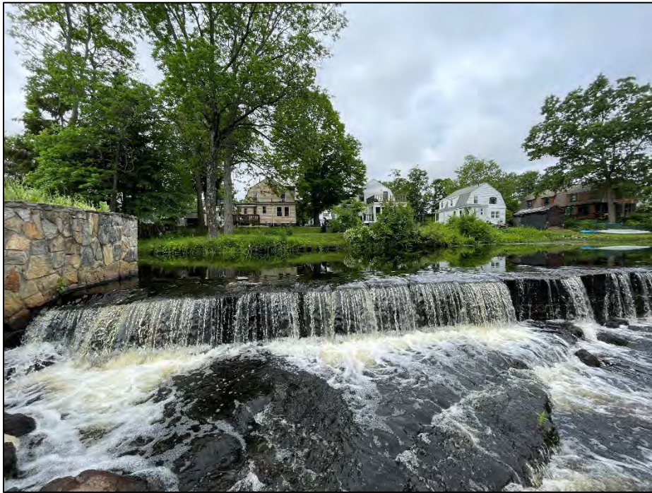
Photo No. 13.: Primary spillway near the right training wall.
