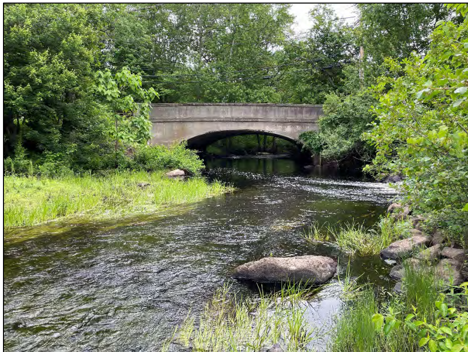
Photo No. 22.: Downstream channel from the embankment between spillways looking towards the Commonwealth Ave. culvert
