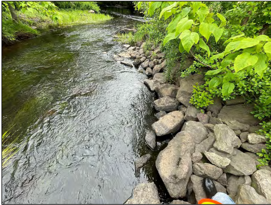
Photo No. 9.: Downstream toe of embankment between the spillway
