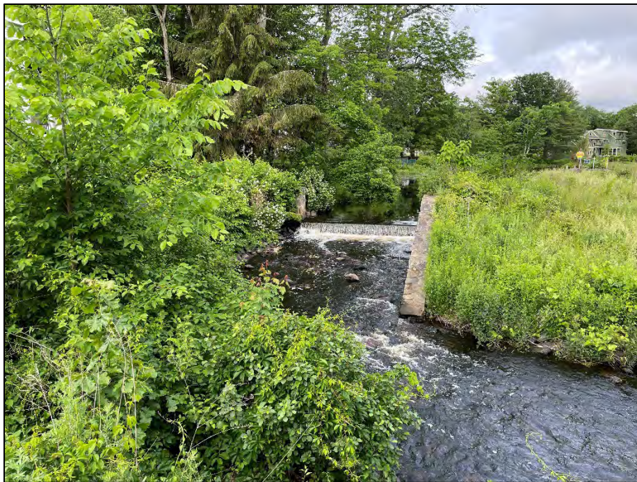
Photo No. 20.: Overview of the downstream side of the auxiliary spillway.
