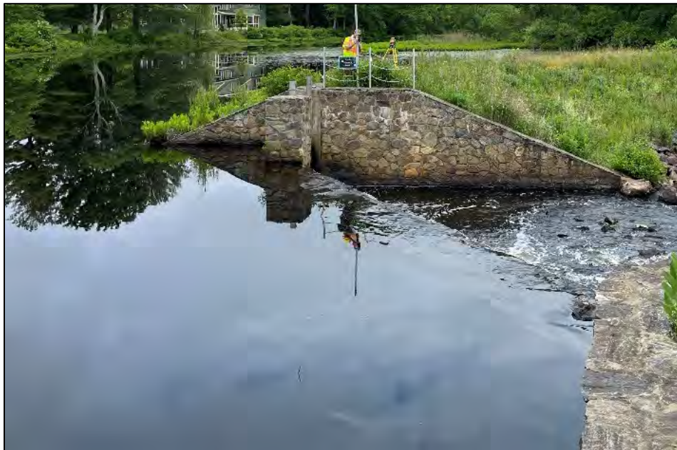
Photo No. 10.: Approach to the primary spillway
