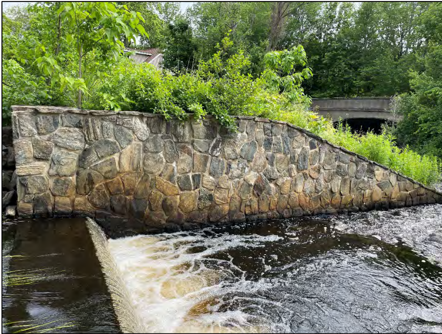
Photo No. 19.: Auxiliary spillway left training wall
