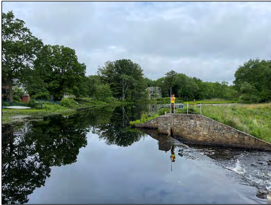
Photo No. 1.: Overview of the impoundment from the auxiliary spillway looking upstream and left
