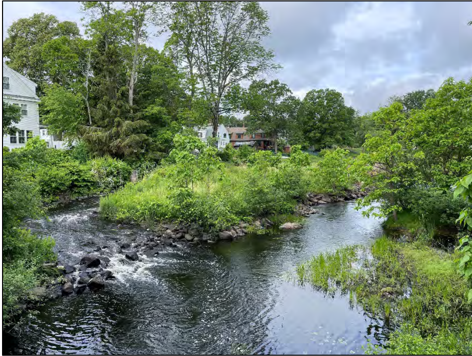
Photo No. 7.: Overview of the embankment between the spillways
