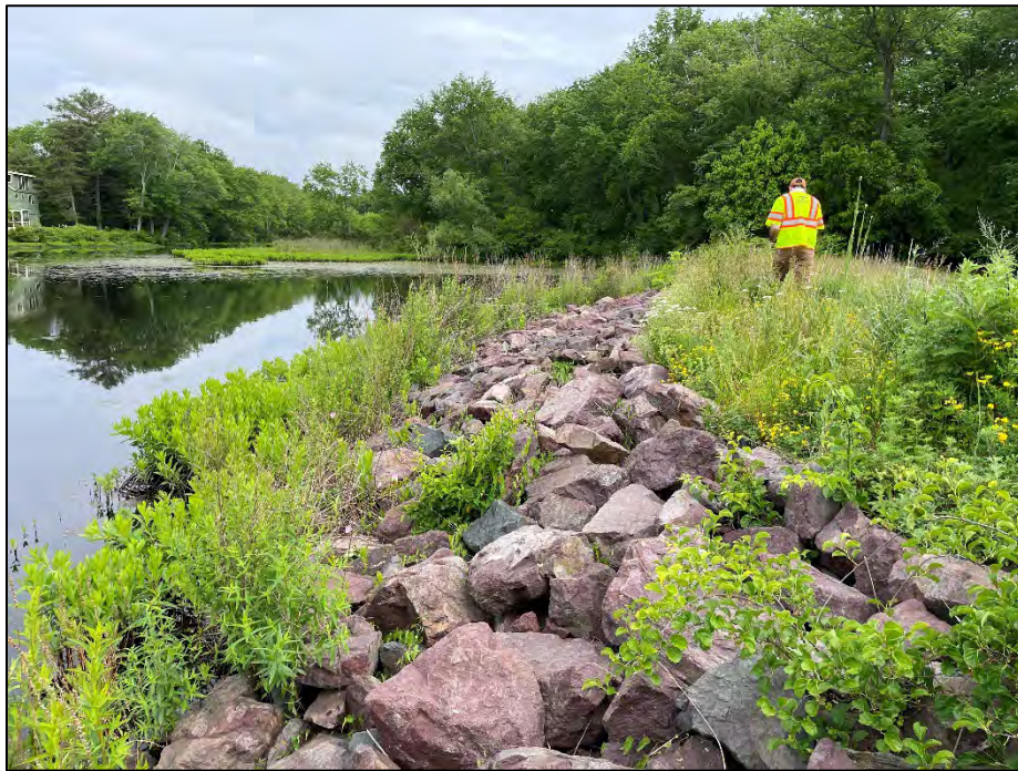
Photo No. 2.: Upstream slope near 1+30 looking left.
