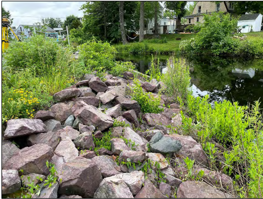
Photo No. 3.: Upstream slope near 1+30 looking right
