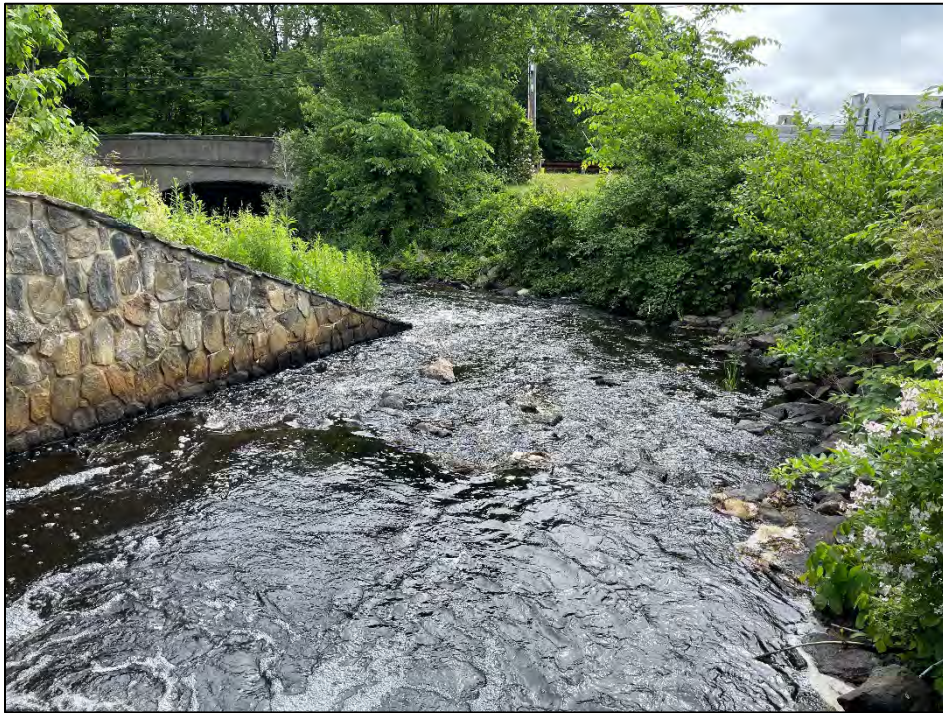
Photo No. 21.: Downstream channel of the auxiliary spillway.
