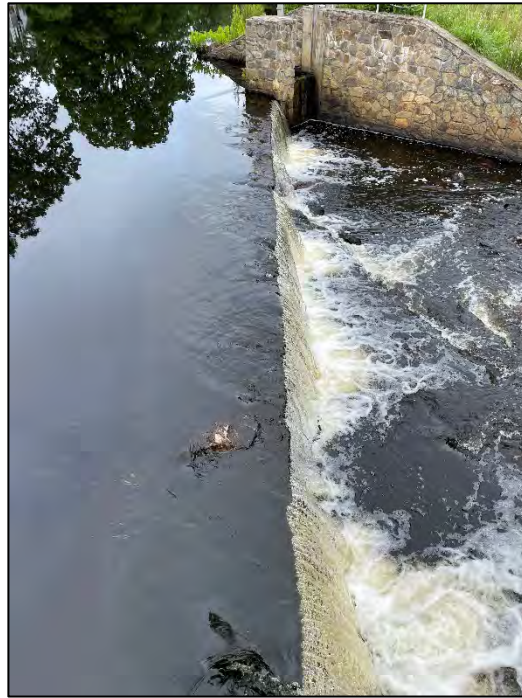
Photo No. 11.: Primary spillway crest from the left training wall.
