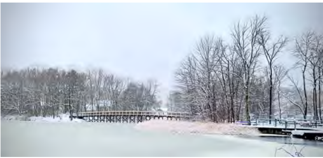
RiverWalk Bridge, photo credit: The Town of Ashland.
