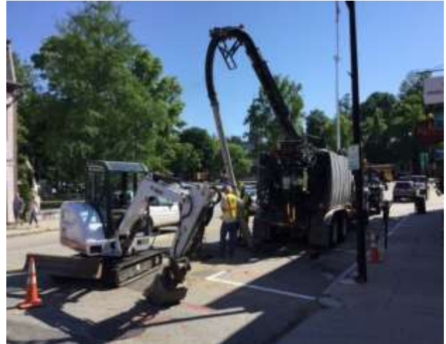
Sewer Main Repair – Main Street
