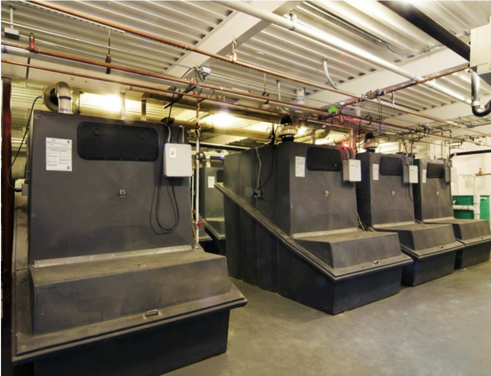
Basement for Composting Tanks
