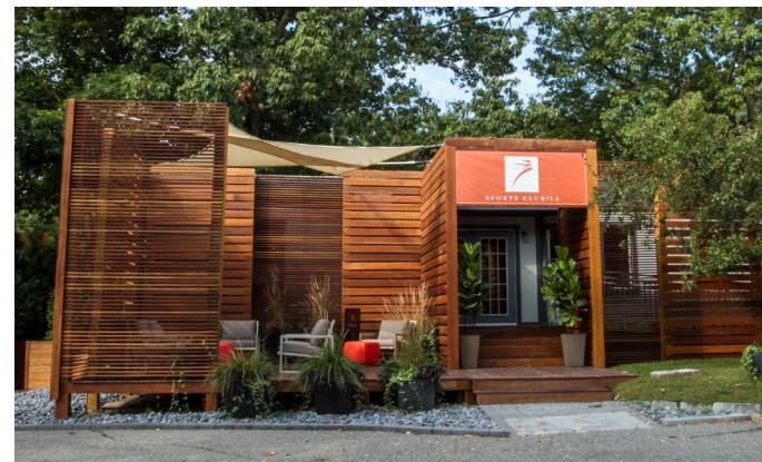
Deck and wood screens
