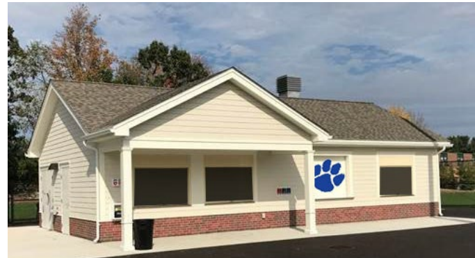
Wood Frame / Siding
