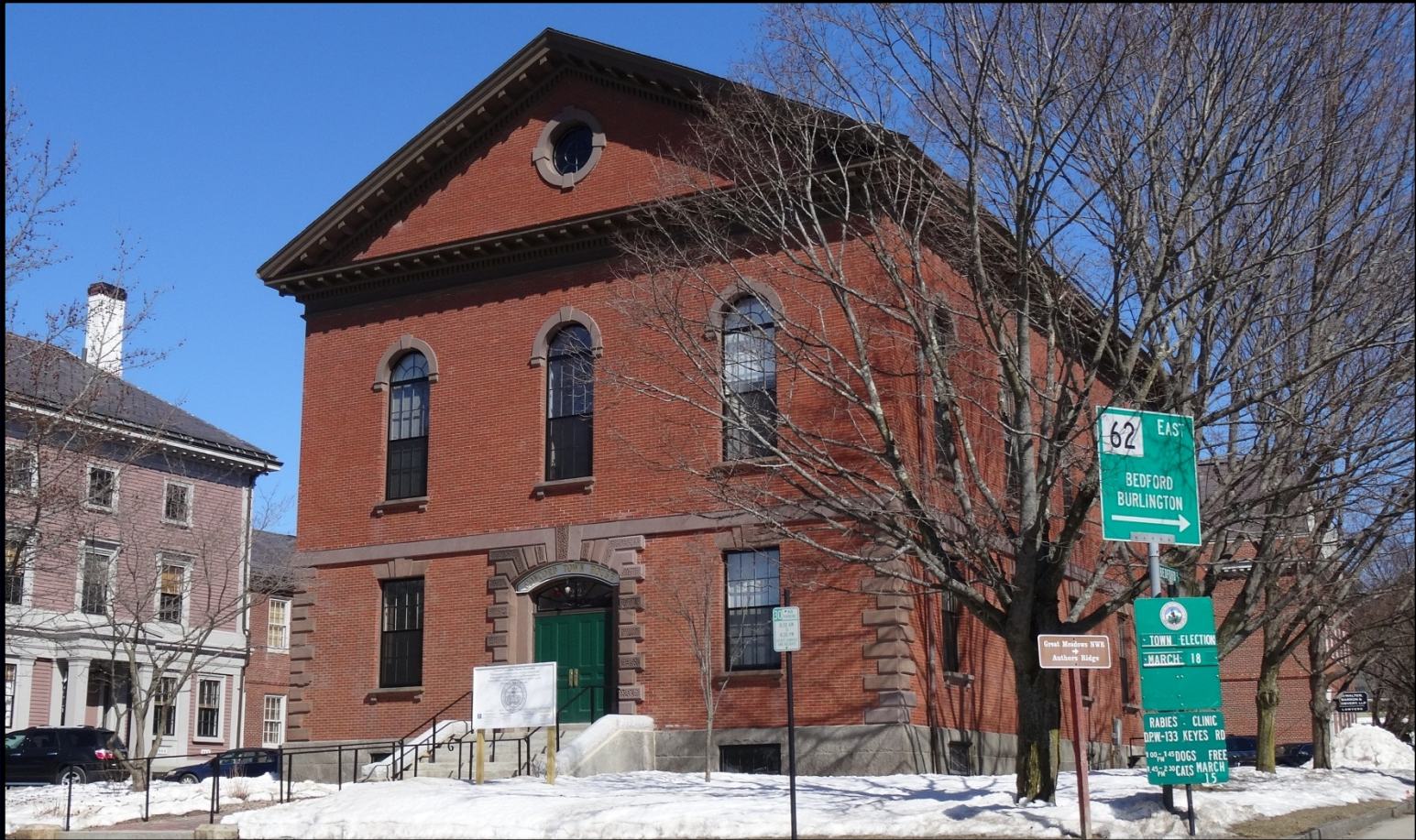
Town House Exterior Restoration (2013)
