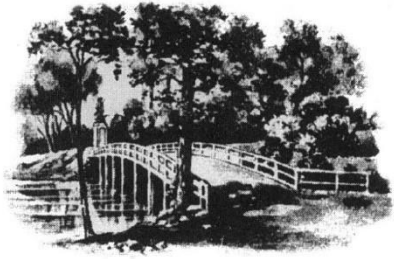
OLD NORTH BRIDGE
