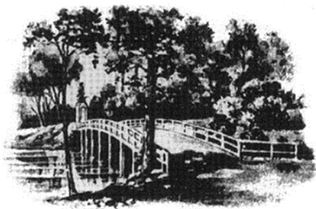
OLD NORTH BRIDGE
