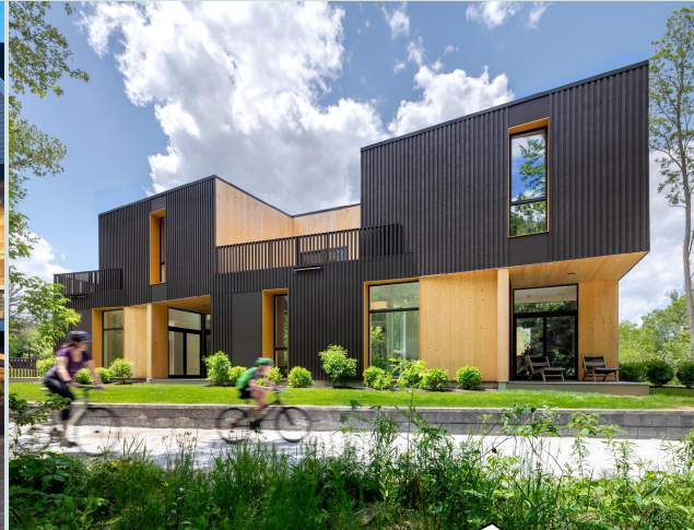
Cable Mills River Houses 14 Units 4.5 Units/ Acre
