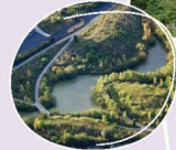
Showcasing Water Infrastructure Systems Lake Whiskey Water Treatment Facility
