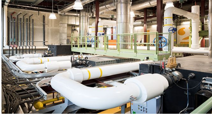
False Creek Neighborhood in Vancouver, BC Sewer Heat Recovery System
