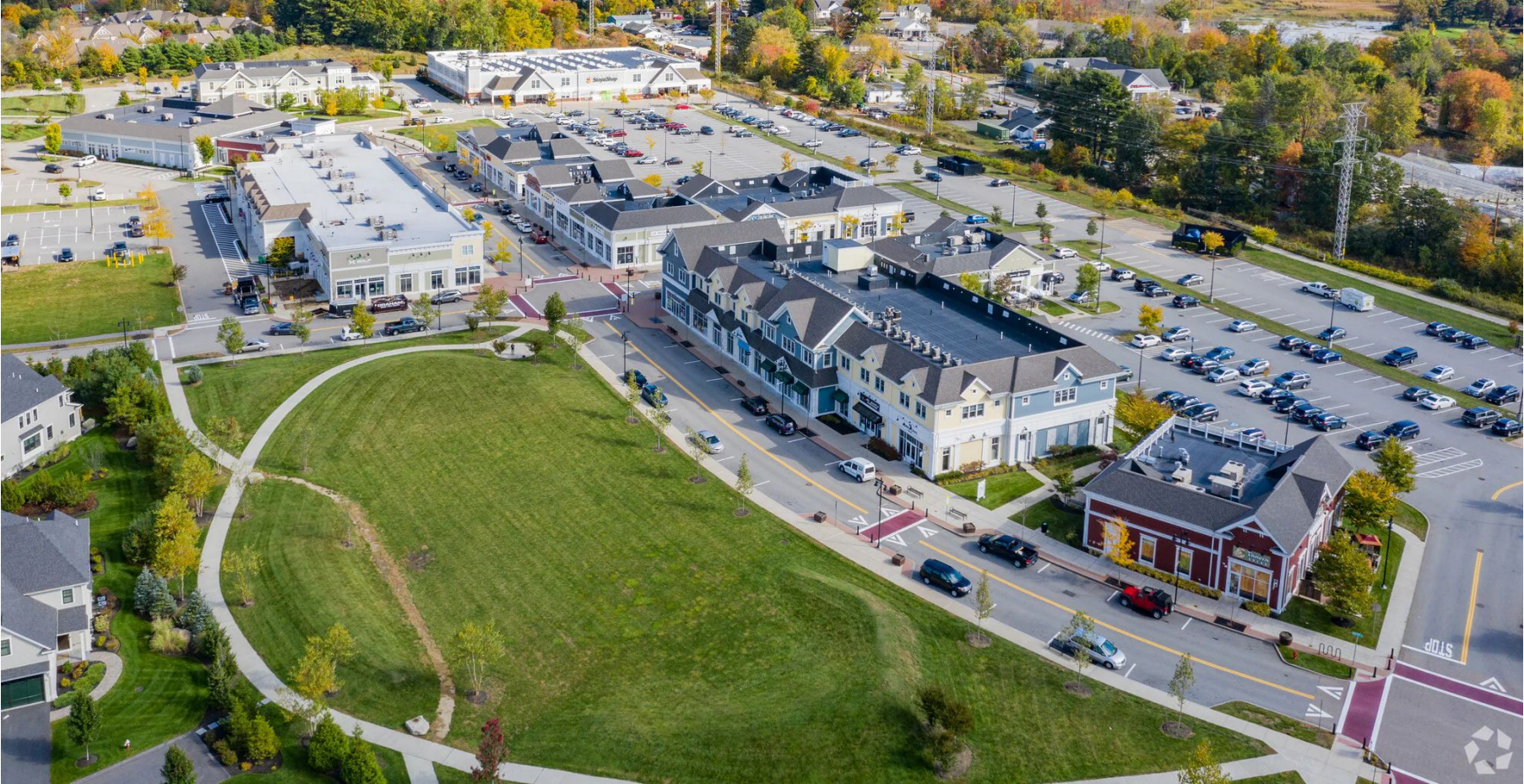
Wayland Town Center, Wayland, MA 52-acre former Raytheon office building > residential, retail & office space, future municipal building, two-acre public green
