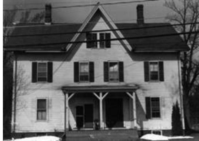
Massachusetts Historical Commission Cultural Resource Concord Reformatory Worker Housing 431 Commonwealth Avenue, Concord, MA Historic Significance: Architectural Style (Victorian) Built: 1878
