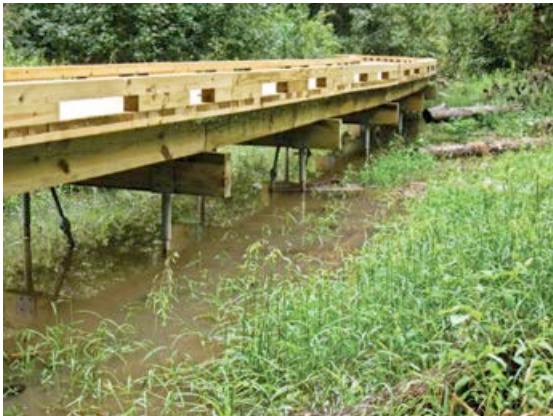
c) Promotional photo from helical pier installer
