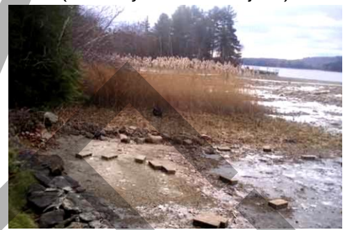
Benthic barrier laid during drawdown over previously cut Phragmites and left for the growing season (above) leading to minimal Phragmites growth the next year (below); untreated Phragmites remains in the background with a cut area ready for barrier deployment in between (Courtesy of Paul Grosjean)
