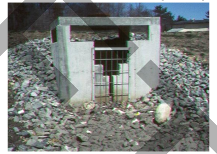
Dry detention basin (above) and flow control outlet (below)
