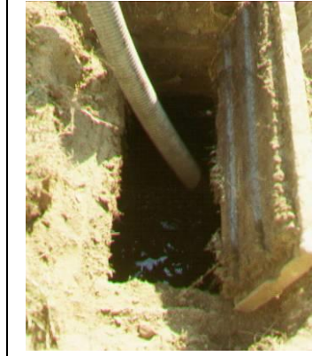
Septic system pump-out
