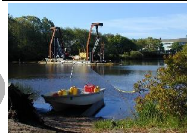
Equipment for reverse layering on Lake Elizabeth (courtesy of Red Lily Pond Protective Association)
