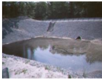
Wet detention basin
