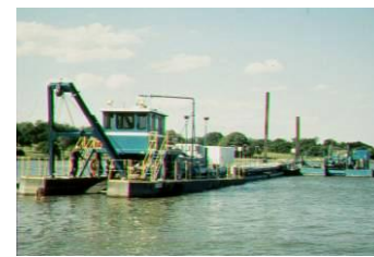
Hydraulic dredging: large cutterhead barge
