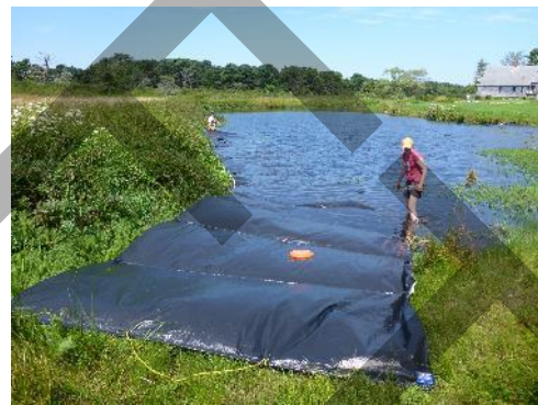
Benthic barrier used to suppress invasive species along shoreline and in shallow water
