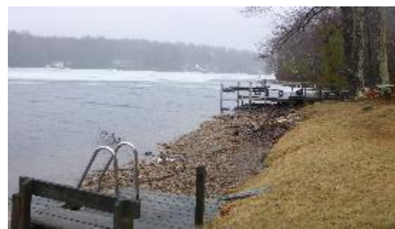
Refill from drawdown in progress
