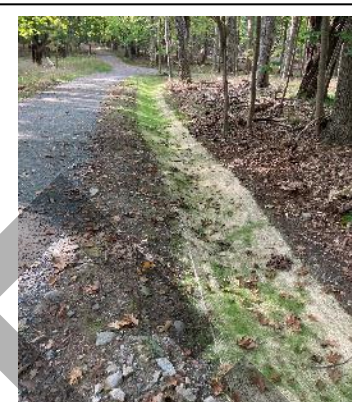
Newly established swale with stabilization mesh supporting vegetation growth
