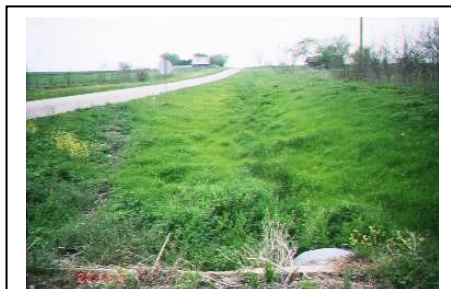
Roadside, vegetated swale
