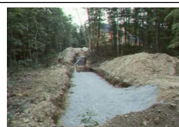
Septic system leachfield being installed
