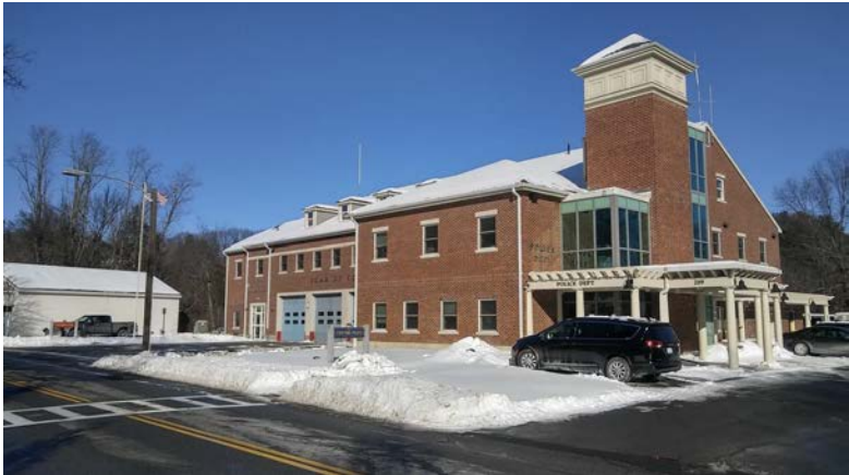
Walden Street Public Safety Campus, Police Station, 219 Walden Street
