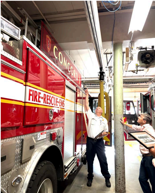
Walden Street, Ceiling height too low for newest trucks
