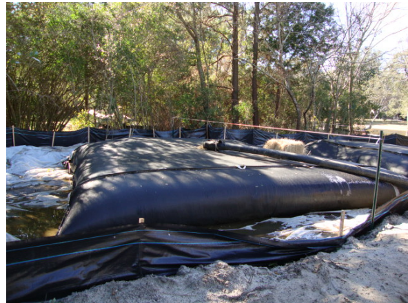
Geotubes used to dewater hydraulically dredged material
