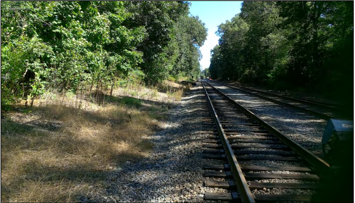
Overview of railroad tracks within MBTA Right of Way.
